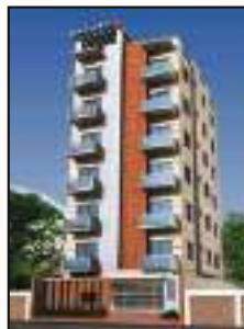
CONCRETE RANGON AYAN
