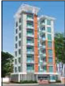
CONCRETE COTTAGE LAKE SIDE
