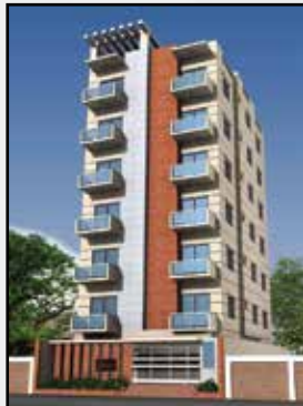
CONCRETE RANGON AYAN
